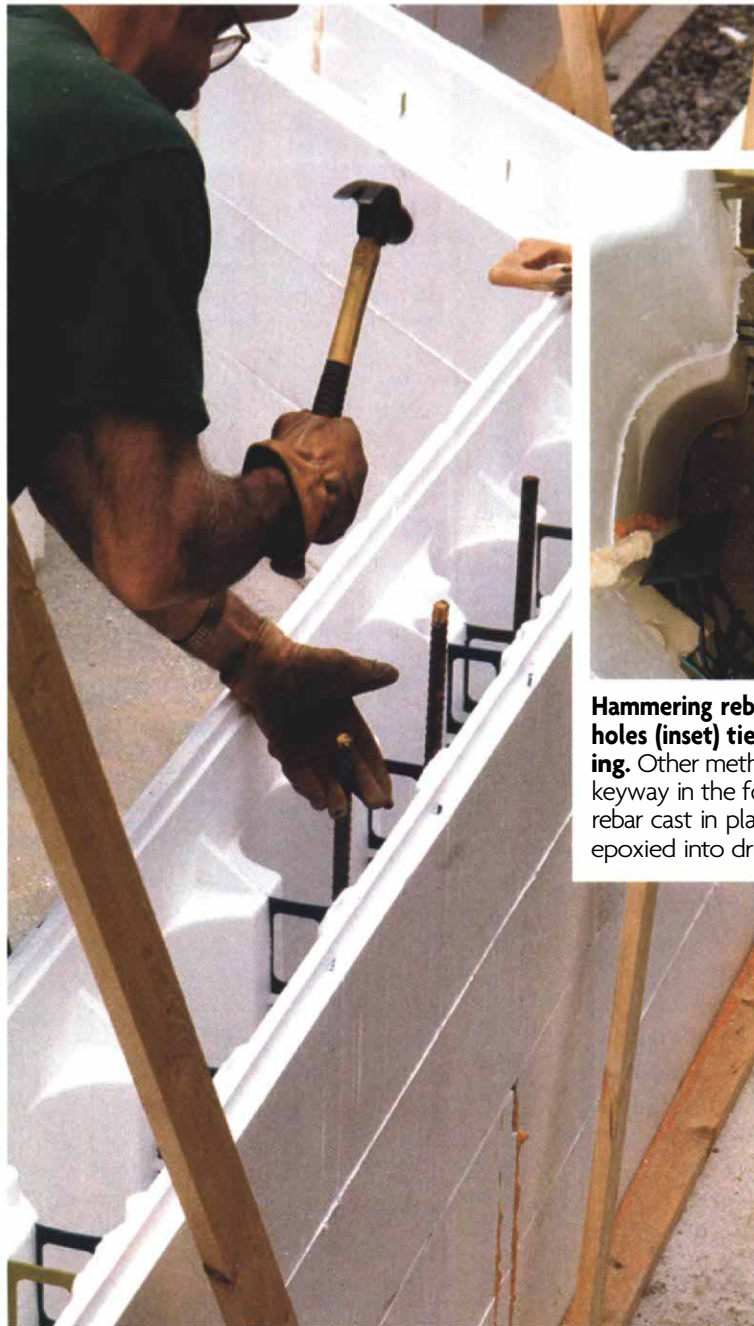
A cleat holds the bottom course in place. It also reinforces the forms in the area subject to the greatest pressure during the pour.
