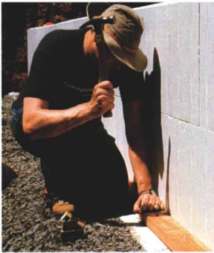
A cleat holds the bottom course in place. It also reinforces the forms in the area subject to the greatest pressure during the pour.
