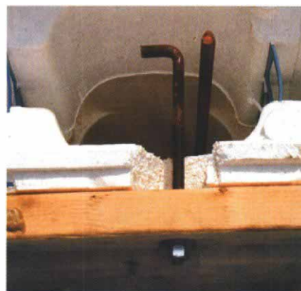
In one variation, steel joists are set and encased in concrete (left). Supported below on a ledger, the floor is sheathed and provides a work platform for pouring walls. In another variation (right), bolts support a ledger. Forms are cut to bring concrete to the ledger, providing a surface for bolts to pinch the ledger against.
