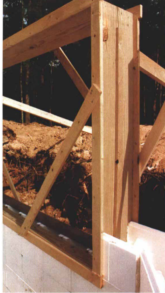
Diagonal braces hold pressure-treated window bucks square. Flanges capture and reinforce cut-to-fit ICFs. Wood strips on the legs will key into the concrete. Kickers and turnbuckles (photo right) hold bucks plumb for the pour.
