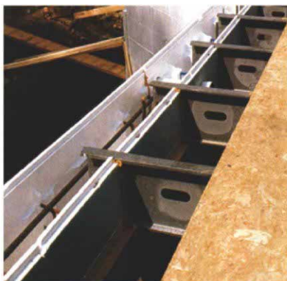
In one variation, steel joists are set and encased in concrete (left). Supported below on a ledger, the floor is sheathed and provides a work platform for pouring walls. In another variation (right), bolts support a ledger. Forms are cut to bring concrete to the ledger, providing a surface for bolts to pinch the ledger against.
