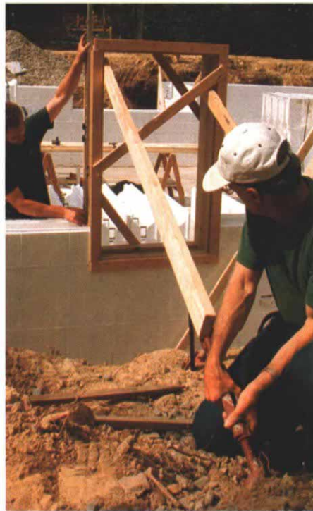
Diagonal braces hold pressure-treated window bucks square. Flanges capture and reinforce cut-to-fit ICFs. Wood strips on the legs will key into the concrete. Kickers and turnbuckles (photo right) hold bucks plumb for the pour.
