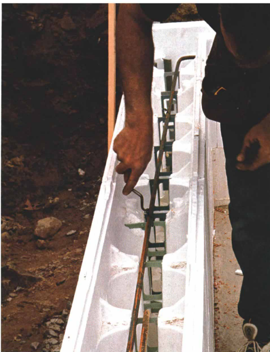
Horizontal rebar is placed in block and plank ICFs as each course stacks. With panel systems, horizontal rebar slides in from the wall ends. With all systems, vertical rebar is placed from above after the top course is set.
